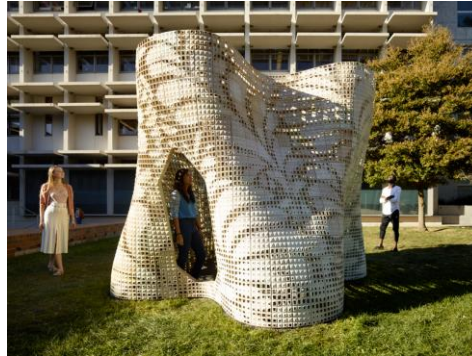
Fig. 3. Example of using cementitious materials to 3D print complex architectural structure, [31]
