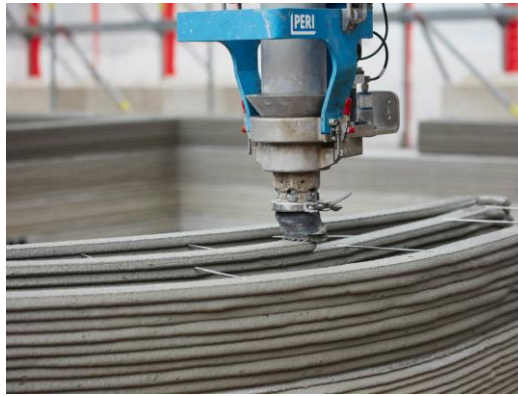
Fig. 5. 3D concrete printing technology [37]
