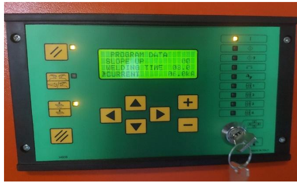
Fig. 2. Digital display of the control panel
